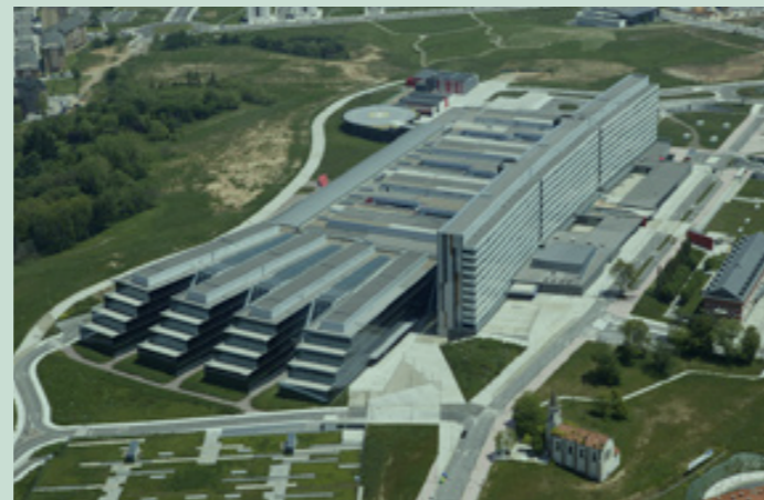
HOSPITAL UNIVERSITARIO CENTRAL DE ASTURIAS Asturias (Spain)
